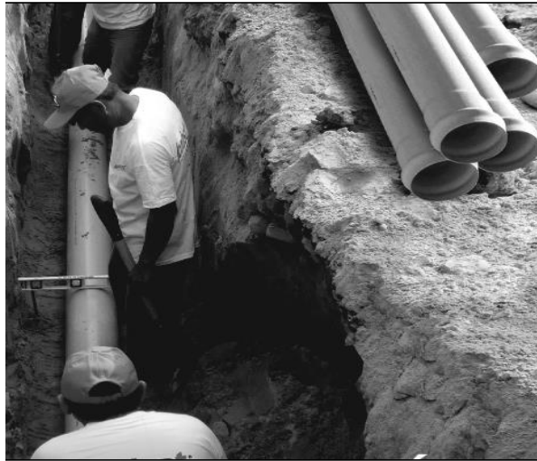
Figure 2. Water networks construction in El Pedregal.
