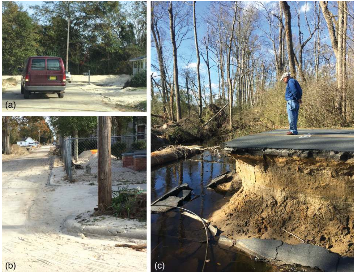
Figure 7. Photos of Robeson County, NC in the months following Hurricane Matthew reveal the extent of sediment transport and deposition by the Lumbee River and damage to local infrastructure by flooding. Sand deposits remained along streets and yards in low-lying parts of Lumberton, Robeson County’s largest town, several weeks after the storm (a, b). Flooding destroyed bridges and culverts throughout the Lumbee River watershed, closing some local roads for months after the storm (c).
